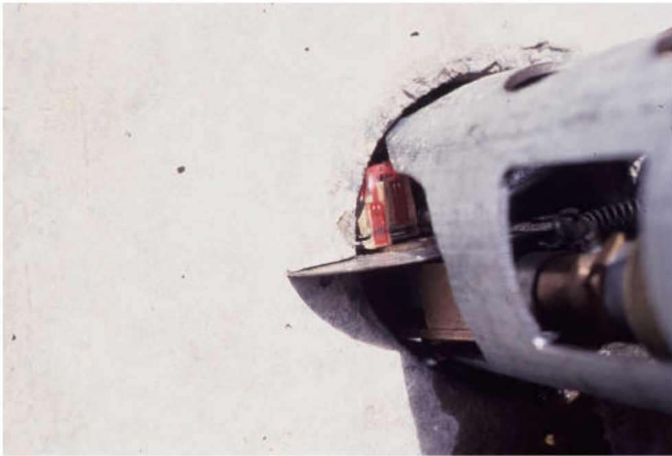
Fig. 1 Borehole slotter at the end of the borehole
